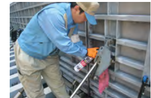
Inspection and repair of flood barriers
