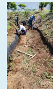
Constructing the walking path
